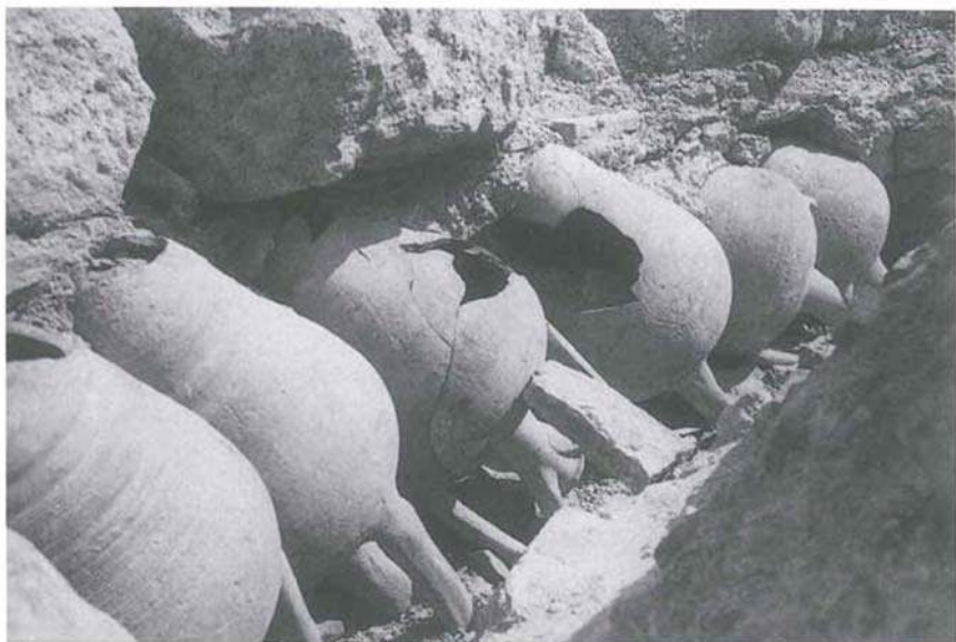
Figure 3. Zeyrek Camii, north church, amphorae at the base of the apse semidome (Z. Ahunbay, 1998).
